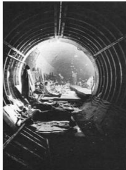
Tube becomes shelter – tracks on the Central line east of Liverpool Street Station filled in with tarmac to accommodate more people.
