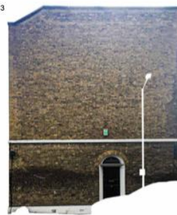
Examples of solid wall London Stock Brick Architecture Georgian Terraces of Bedford Square (2), Sidney Square (3)
