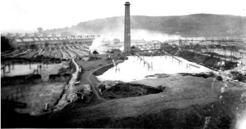
Whickham Lane Brick Fields in Plumstead: 1901. The image shows the typical organisation of quarry and construction site sharing the same site and being operated simultaneously same to formulate the local vernacular of brick terraces. Photograph - Gibbs A., 1901, Whickham Lane Brickfields. Available at: http://www.plumstead-stories.com/ (Accessed 21 January 2022)
