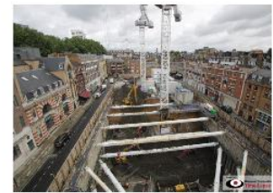
Marylebone Square basement excavation ( https://its.time-lapse-systems.co.uk/viewer/klar-marylebone-square-c042021/ )
