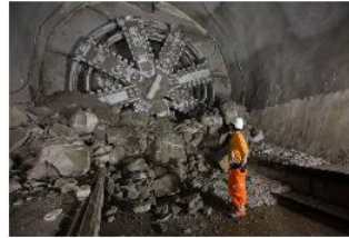
Crossrail Boring ( https://www.theconstructionindex.co.uk/assets/2020/ )
