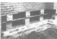
Underpinning with Pyleford studs
